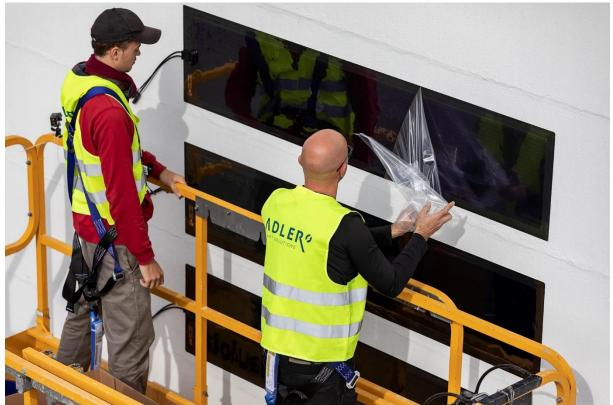
Caption 3: With the help of the integrated adhesive on the back, the HeliaSol® solar films can be precisely attached by the assembly team.
